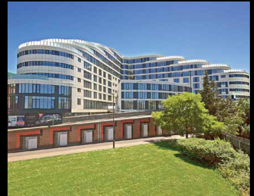
Bradstowe House, Harrow, Middlesex, London
